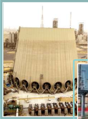
Cooling Tower 200 Ton refrigeration
